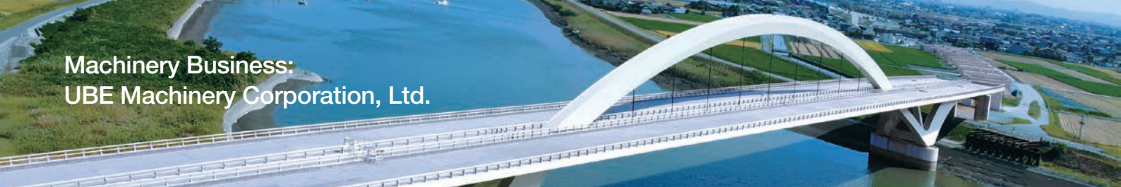
Hayatsue River Bridge
