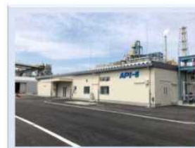
Fifth pharmaceutical plant
