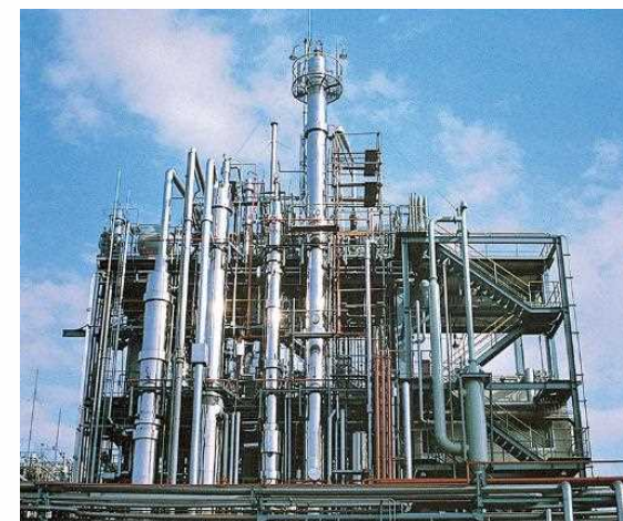
DMC manufacturing facility (Japan)
