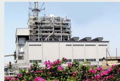
IPP power plant
