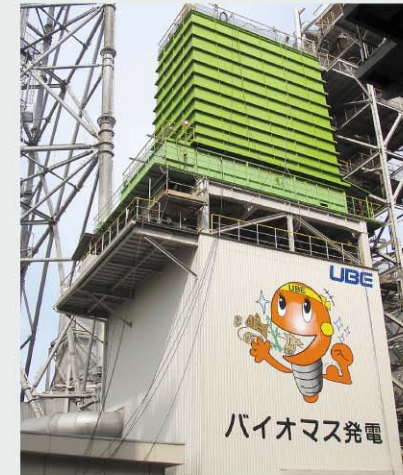
Biomass fuel facility
