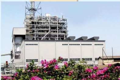
IPP power plant
