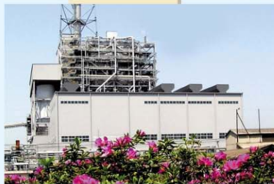
IPP power plant
