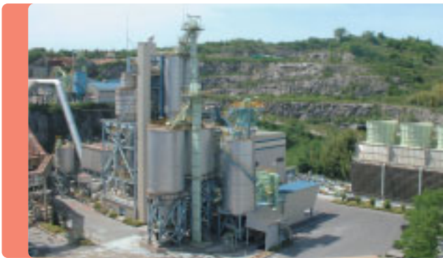
Coal/woody biomass-mix power generating facilities
