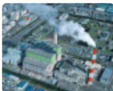
Incinerator using Calbreed SII and Solbalit
