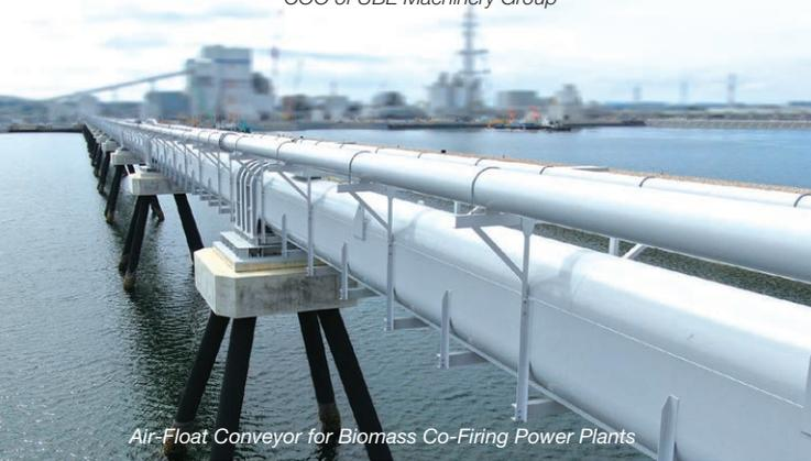
*Air-Float Conveyor for Biomass Co-Firing Power Plants*
