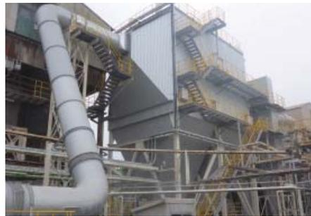
Electrostatic precipitator (Ube Material Industries, Ltd.)
